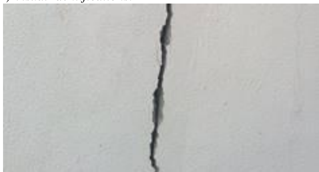
Fig 1. Crack on the wall Width: Above 5mm Type: Wide Crack Probable Cause: Thermal Variation
