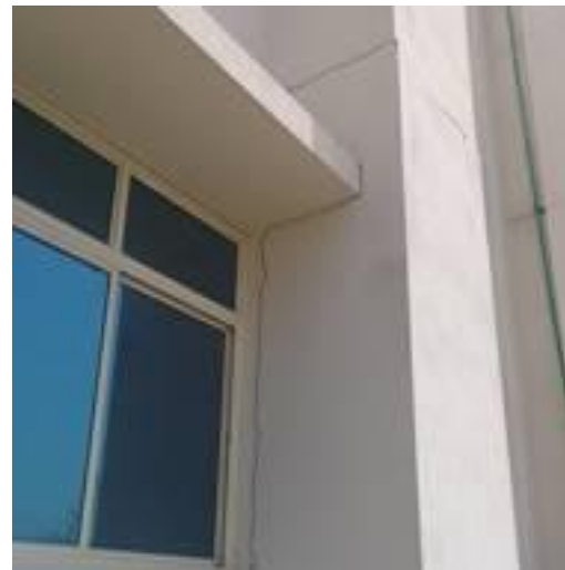
Fig. 4. Crack above window Width: Between 1 to 2mm Type: Medium Crack Probable Cause: Shrinkage
