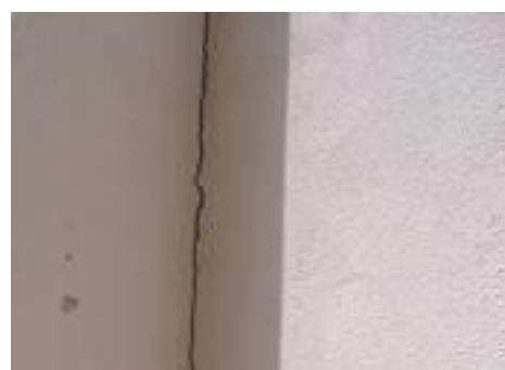
Fig. 2. Crack at the corner Width: Above 2mm Type: Wide Crack Probable Causes: Temperature Variation or Shrinkage
