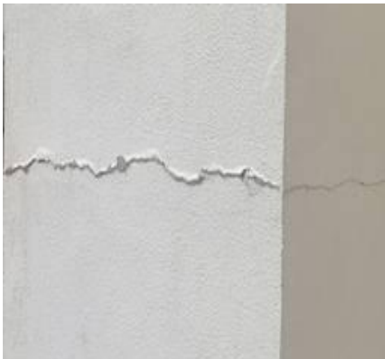
Fig. 3. Horizontal Crack Width: Between 1 to 2mm Type: Medium Crack Probable Cause: Thermal Movement
